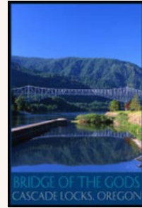
IL-3218 Bridge of the Gods Over the Columbia River
